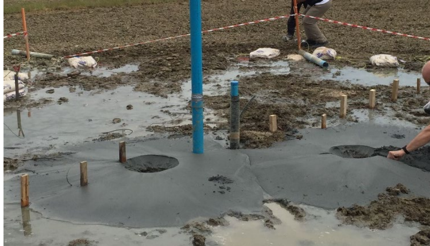
Figure 7.19: Multiple sand boils and ejecta, evidence of liquefaction, observed during blast 1 near the center of the unimproved natural panel (NP).
